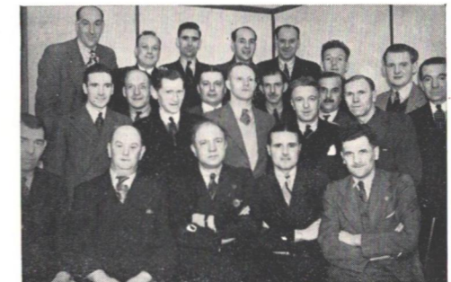
This photograph was taken on the occasion of the official opening of 194 Oxford Street
